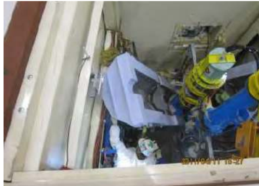
Removal of Pb shield walls 22
